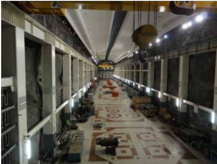
Tala HPP – Powerhouse cavern
