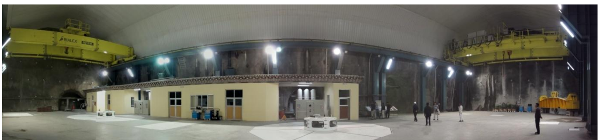
Dagachhu HPP – Powerhouse cavern
